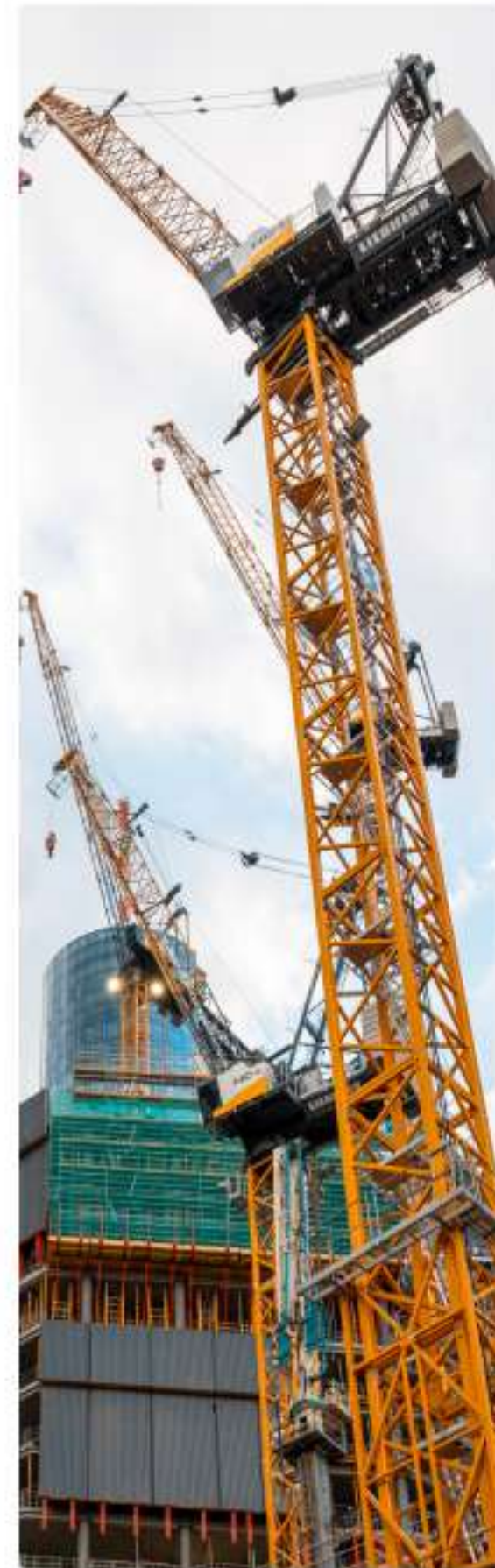
Construction and BMS
